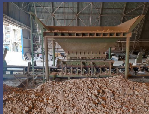
Tolva recepción yeso
